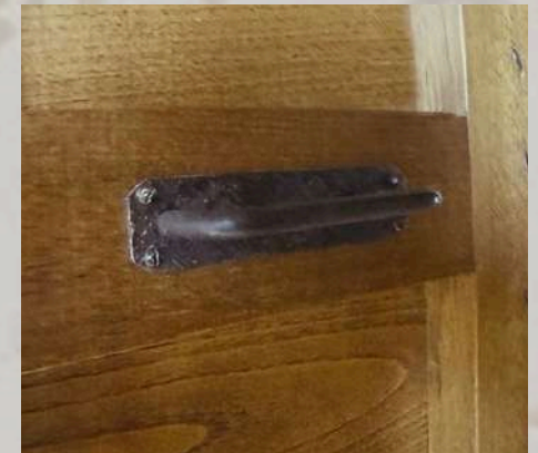
Portellone Mercantile: particolare interno, maniglietta in ferro battuto Board and Batten Shutter: interior detail, wrought iron handle.
